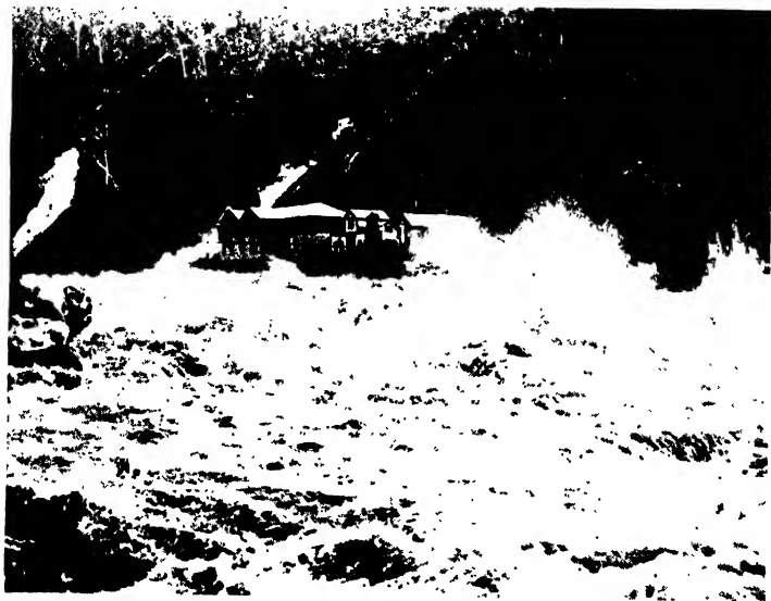
FIG. 101. CATARACT GORGE AND POWER-STATION, NEAR LAUNCESTON By courtesy of the Immigration Office, Commonwealth of Australia
